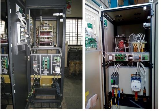
Servo controlled voltage corrector designed for Rishab Industries (Bulk manufactured for Emerson Network Power, Neowatt systems)
